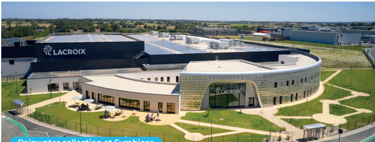
Rainwater collection at Symbiose
